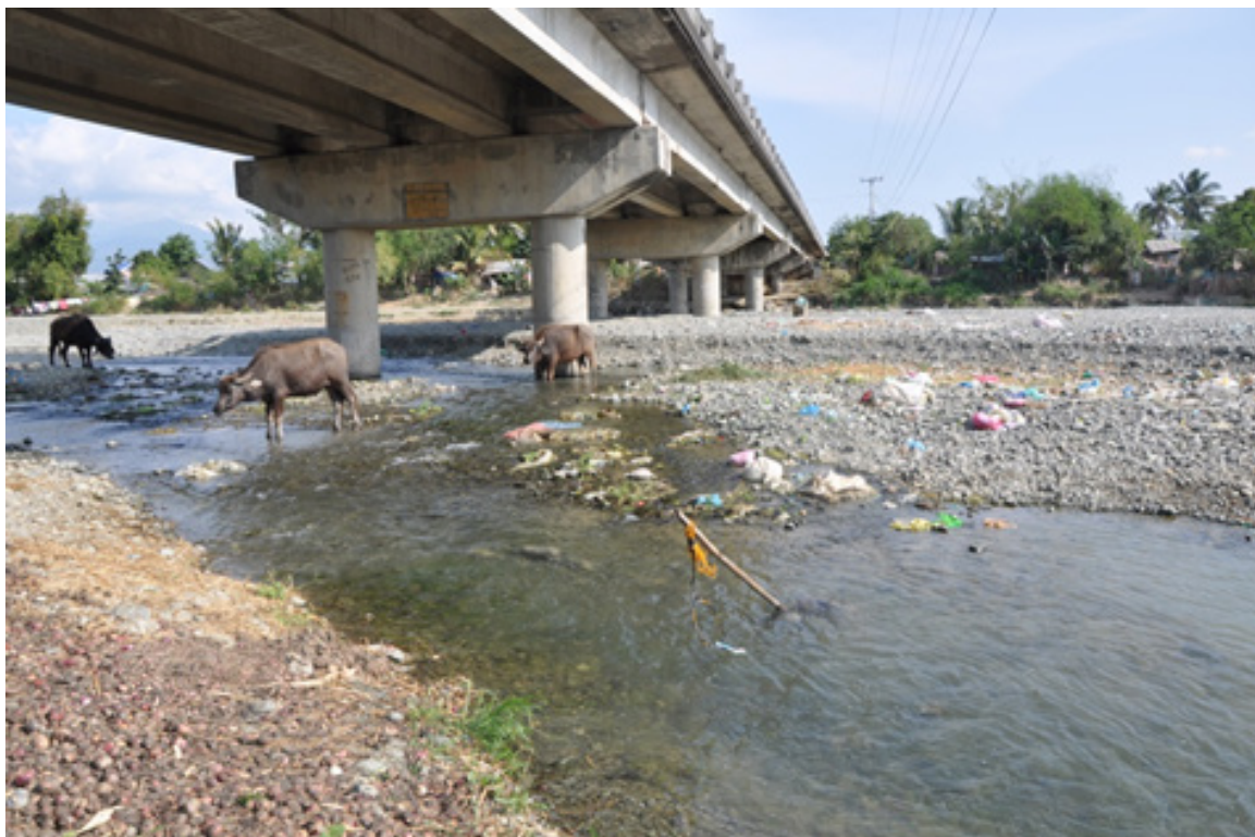
Figure 43. Flow Measurement set up in Vega Bridge-1
