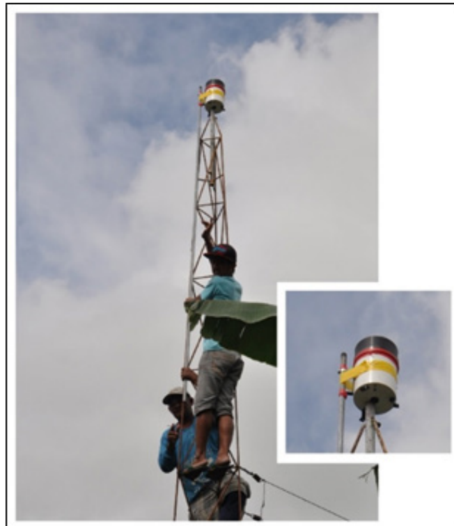
Figure 17. Rain Gauge deployment in Brgy. Barcenaga, Naujan Oriental Mindoro
