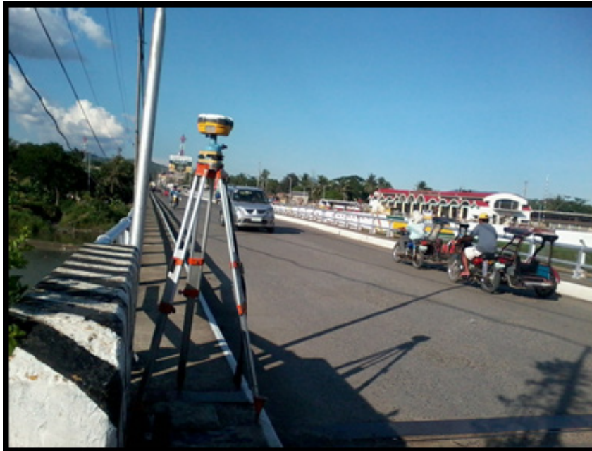
Figure 51: AB – 1 is located in Jalaur Bridge located at Passi City
