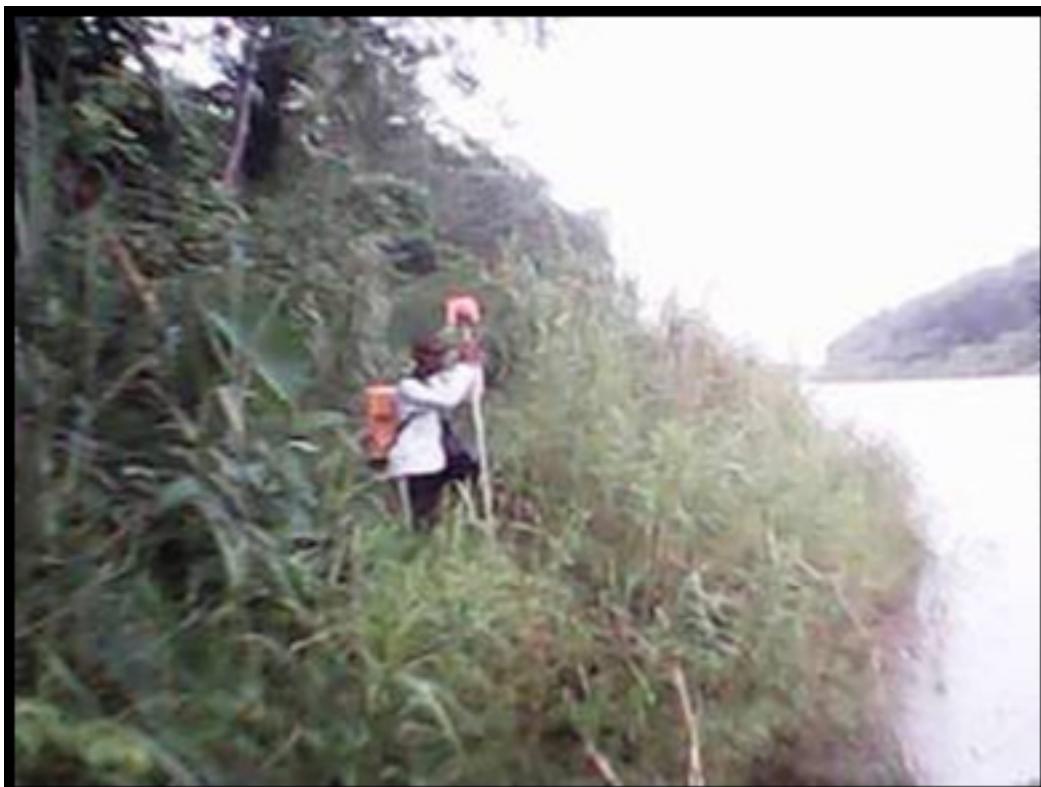
Figure 108: Conducting profile survey using Total Station at Brgy. Panda, Dueñas
