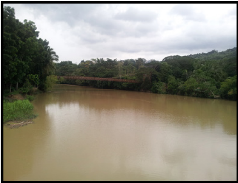
Figure 104: Hanging Bridge near the dam located between Brgy. Licu-an and Brgy. Moroboro, Dingle.
