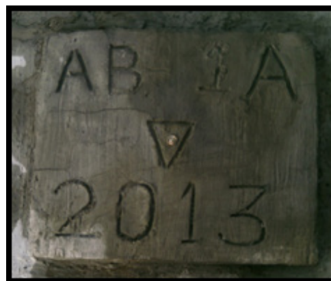
Figure 58: AB – 1A is located in Jalaur Bridge in front of Passi Terminal located at Passi City
