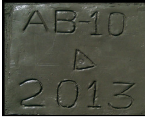
Figure 77: AB – 10 is at Banga-Bante Bridge located at Barangay Balabag, Dumangas
