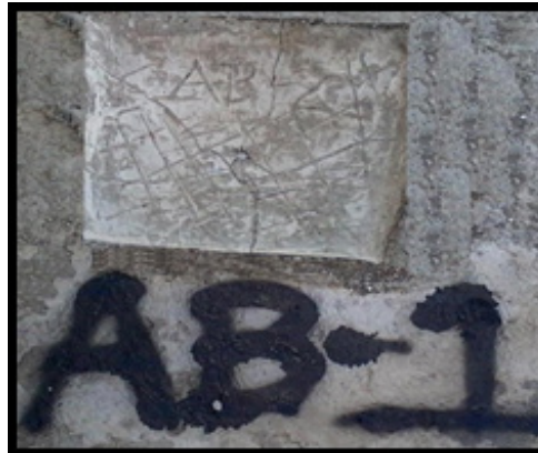
Figure 57: AB – 1 is located in Jalaur Bridge located at Passi City
