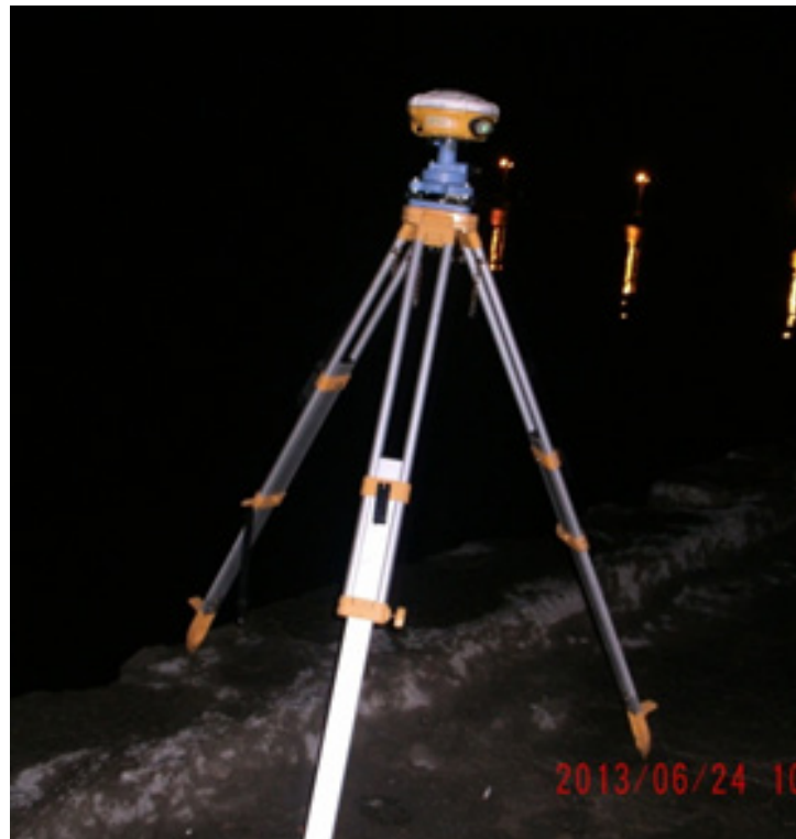
Figure 36. Static GNSS survey at DVS-1 located at Sta Ana wharf, Davao City
