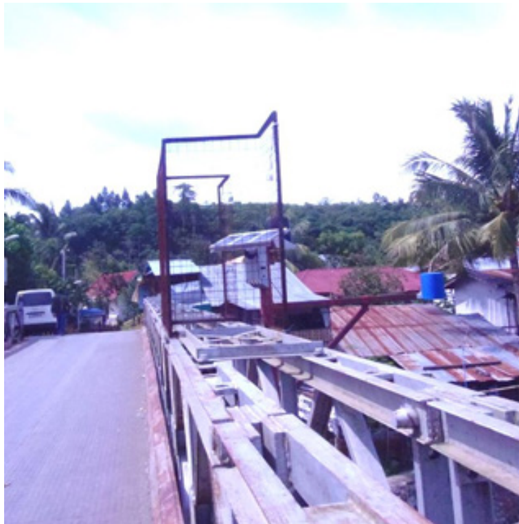
Figure 27. Installed AWLS on Matina Pangí Bridge II
