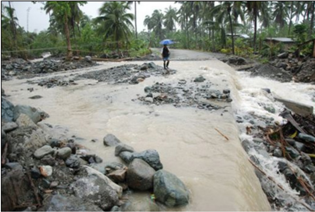
Figure 83. The access roads to the cross-sections drop off points were blocked. Vehicles cannot pass on the area
