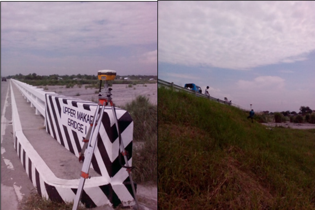
Field verification at Makar River
