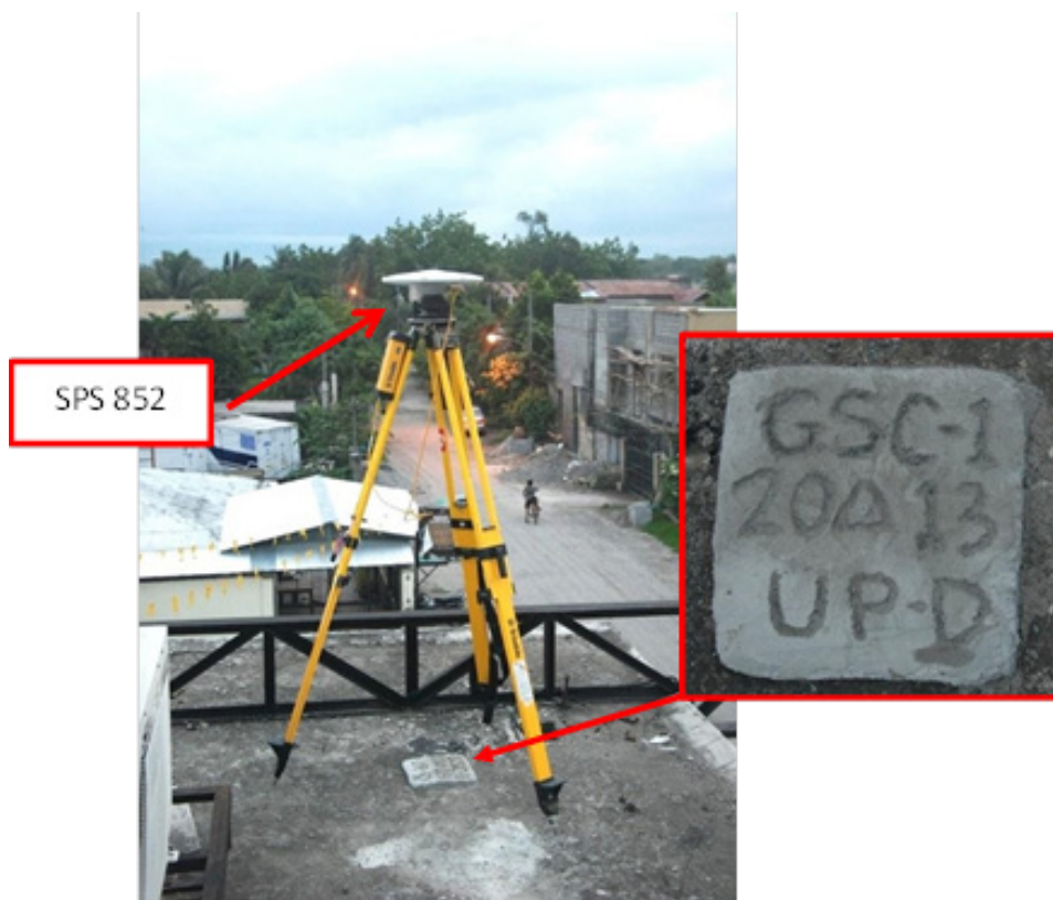
Figure 14. GNSS base station at GSC-1, rooftop of ICE hotel in General Santos City
