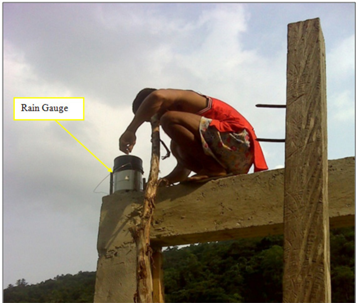
Figure 22. Deployment of rain gauge in Brgy. Batangan, General Nakar
