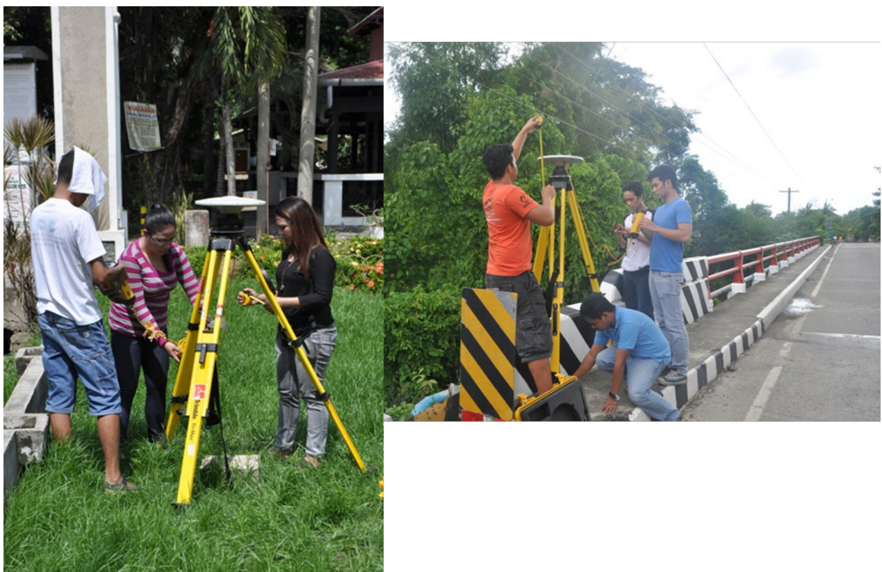
Figure 17. Base Station set-up for Phase 2 of Control Survey in Agno River
