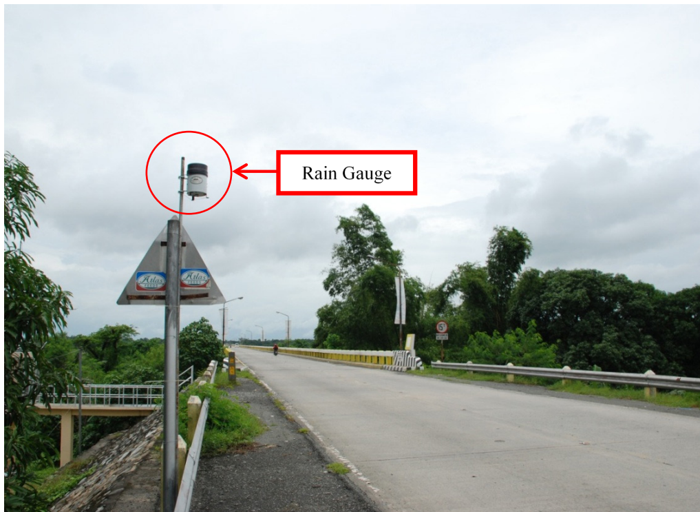
Figure 42. The rain gauge installation on Narciso Ramos Bridge, Bgy. San Patricio, Sta. Maria, Pangasinan
