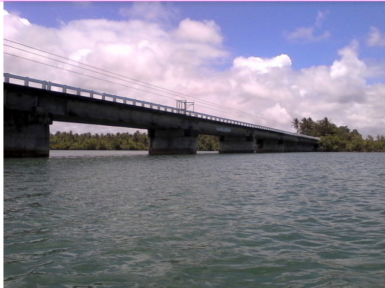
Figure 35. Upstream/downstream side of Can-Avid Bridge
