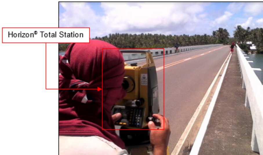
Figure 36. As-built survey of Can-Avid Bridge
