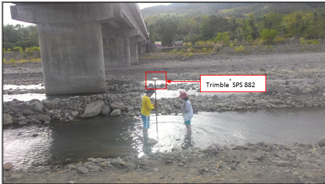
Figure 36. Cross-section survey for the Subangdaku River
