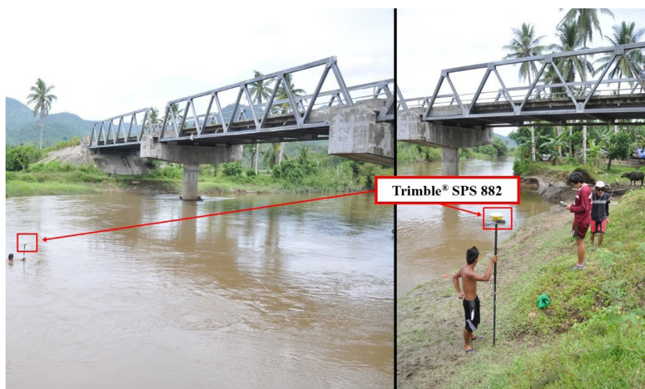
Figure 40. Cross-section survey of Calay-Calay Bridge
