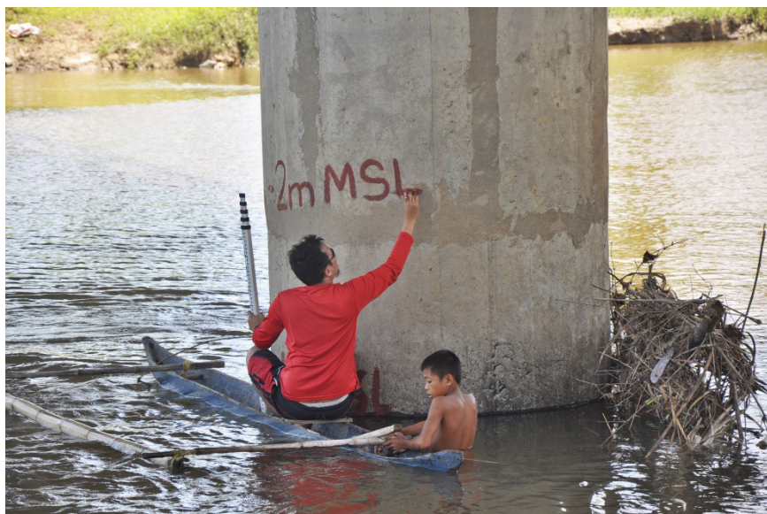
Figure 44. Water-level marking at one of the piers of the Calay-Calay Bridge
