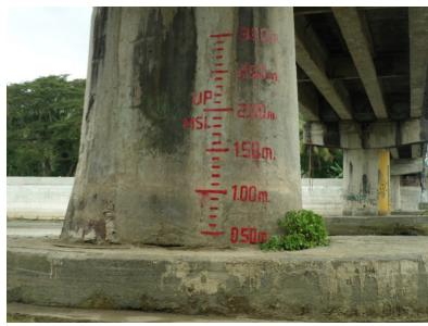
Figure 40. Water level marking at Salug Bridge
