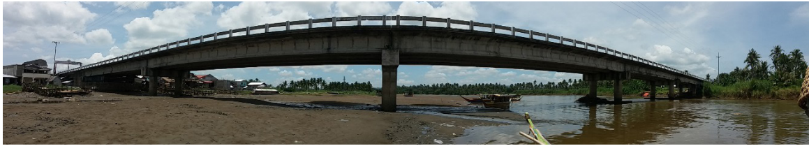
Figure 36. Pambujan Bridge facing upstream.
