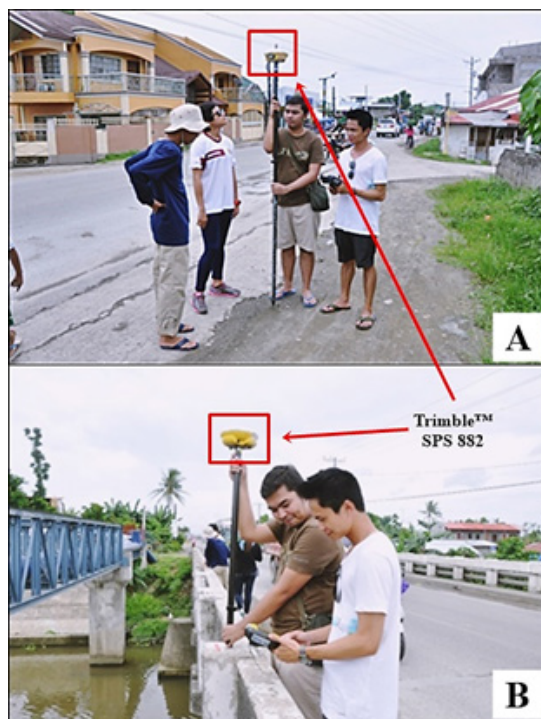
Figure 41. Cross-section survey using Trimble® SPS 882 – (A) bridge approach and (B) bridge deck of Bernard Reed Bridge, Palo, Leyte
