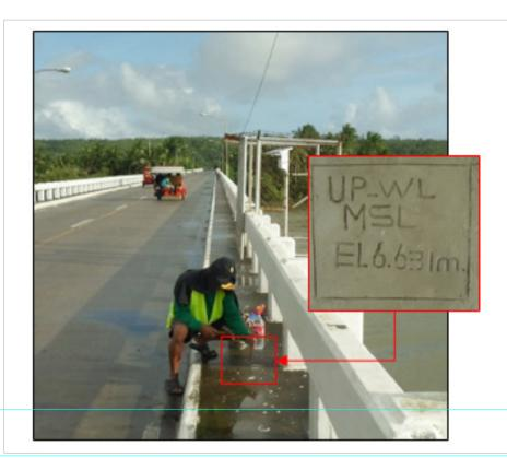
Figure 37. Water surface elevation marking on Oras Bridge sidewalk
