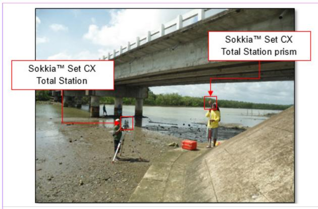
Figure 32. As-built survey of Oras Bridge
