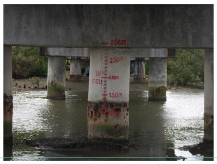
Figure 38. Water level markings on the pier of Oras Bridge
