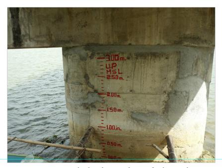
Figure 37. Water level markings on the pier of Dolores Bridge
