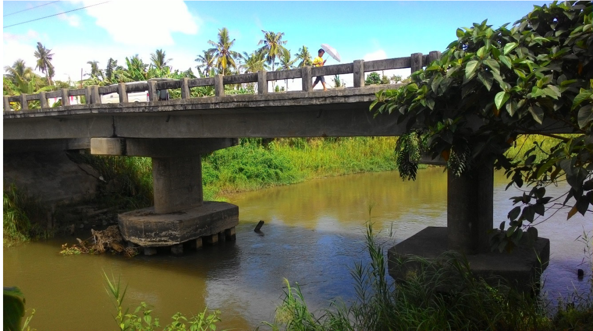
Figure 45. Sta. Elena Bridge facing downstream
