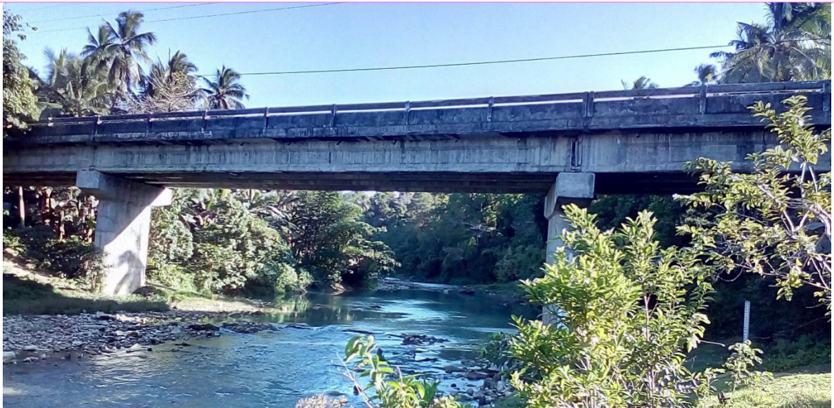
Figure 38. Cambanog Bridge facing downstream
