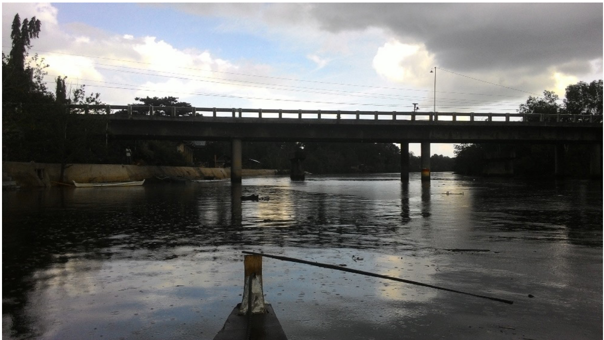
Figure 47. Water-level markings on Trinidad Bridge
