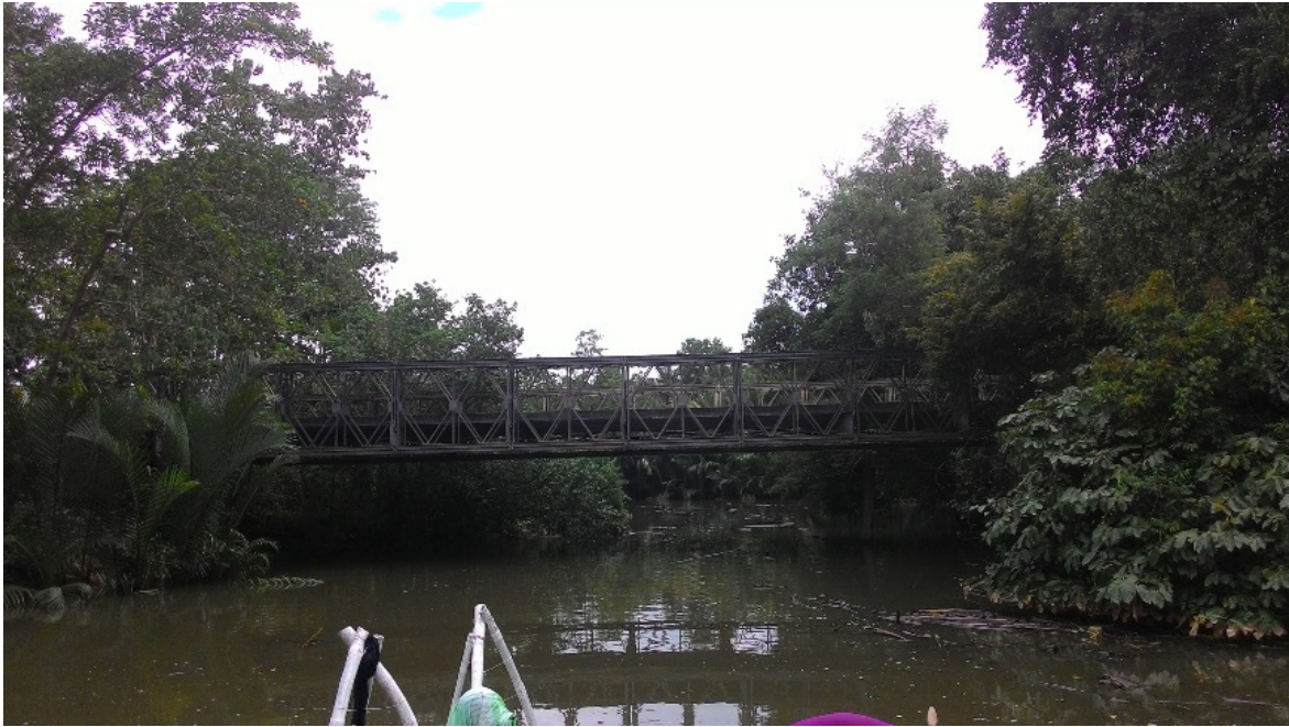
Figure 36. Tugas Bridge facing upstream
