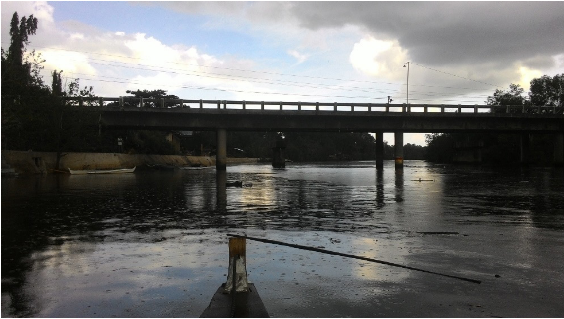
Figure 38. Trinidad Bridge facing downstream
