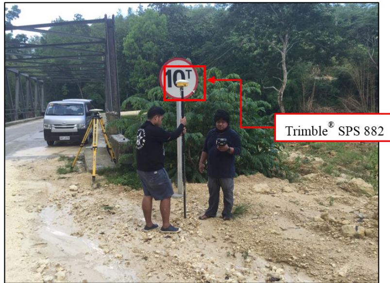
Figure 37. Bridge as-built survey using PPK Technique
