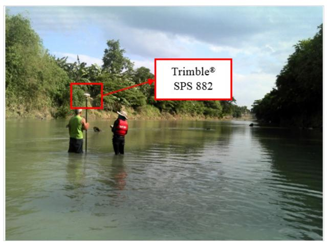
Figure 43. Bathymetric survey setup in Padada-Mainit River (upstream)
