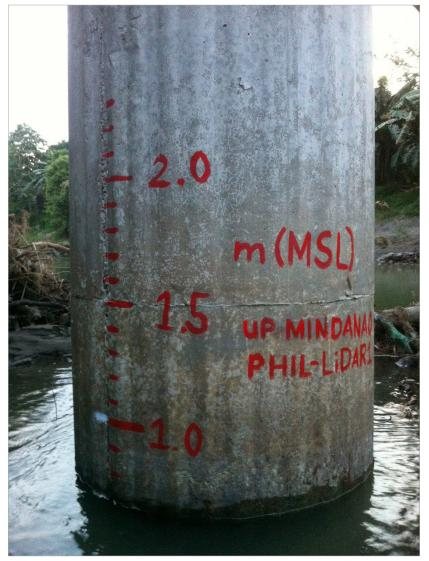
Figure 40. Water level markings on the post of Tologan Bridge
