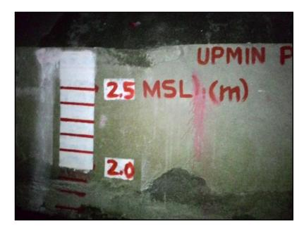
Figure 39. MSL water level markings in Digos Bridge's Pier
