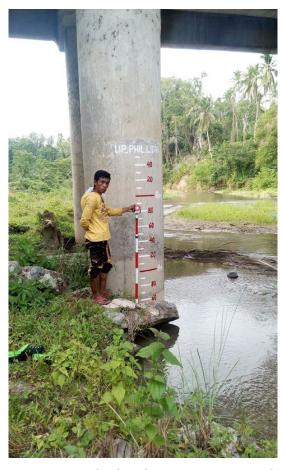
Figure 41. Water-level markings on Bitanagan Bridge
