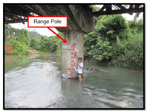
Figure 37. Water-level markings on Ransang Bridge
