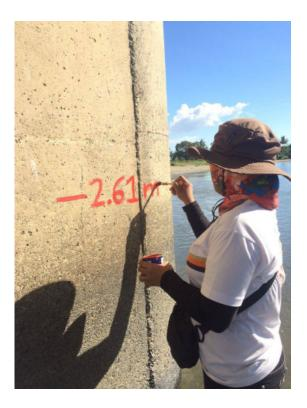
Figure 44. Water level marking at Salagan Bridge, Brgy. Casague, Municipality of Sta. Cruz
