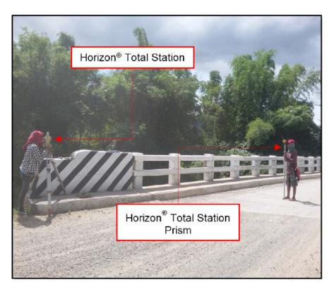
Figure 34. As-built survey of Panitian Bridge
