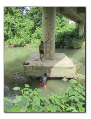
Figure 38. Water-level markings on Panitian Bridge
