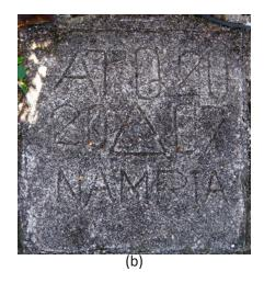
Figure 6. GPS set-up over ATQ-20 as recovered in Brgy. Zaragoza of Bugasong (a) NAMRIA reference point ATQ-20 (b) as recovered by the field team.
