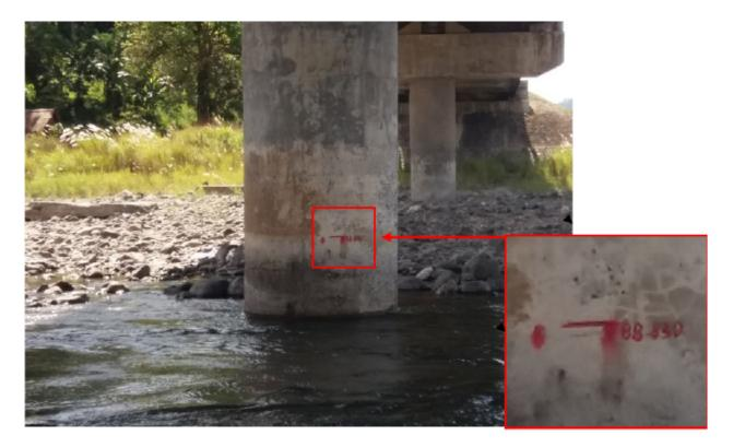
Figure 44. Water-level marking at Mompong Bridge, Brgy. Sta. Lucia, Municipality of Sablayan
