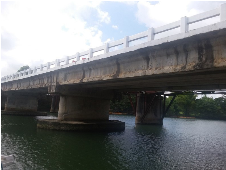
Figure 36. Iwahig Penal Bridge facing upstream
