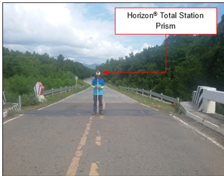
Figure 37. As-built survey of Iwahig Penal Bridge
