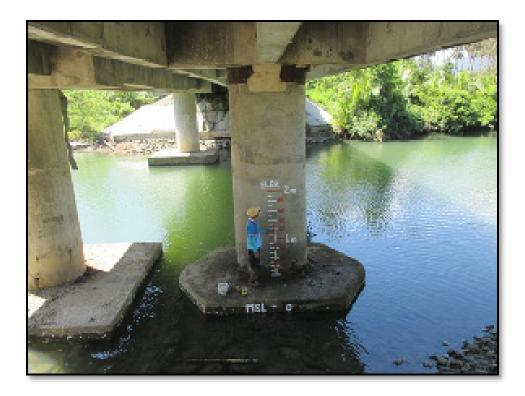
Figure 41. Water-level markings on Inagauan Bridge
