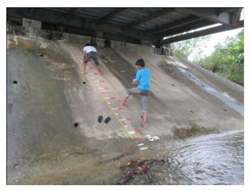
Figure 38. Water-level markings on Ilog-Ilog Bridge.
