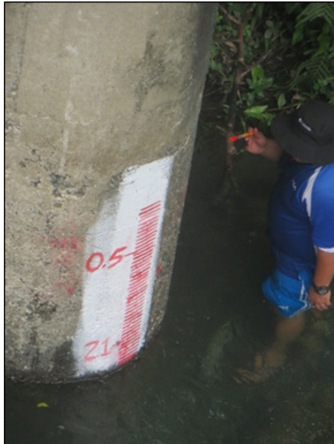
Figure 44. Water level marking on one of Subaan Bridge's pier
