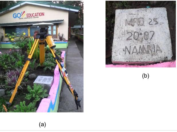
Figure 3. (a) GPS set-up over MRQ-25, at the top of the plant box near the gate of Tugos Elementary School in Barangay Tugos, Boac, Marinduque; and (b) NAMRIA reference point MRQ-25, as recovered by the field team
