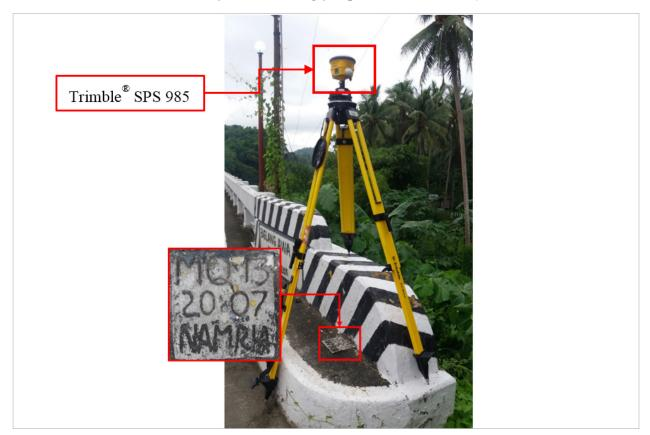
Figure 28. GNSS receiver set-up, Trimble® SPS 985 at MQ-13, located at the approach of the Biglang Awa Bridge in Barangay Mataas na Bayan, Boac, Marinduque
