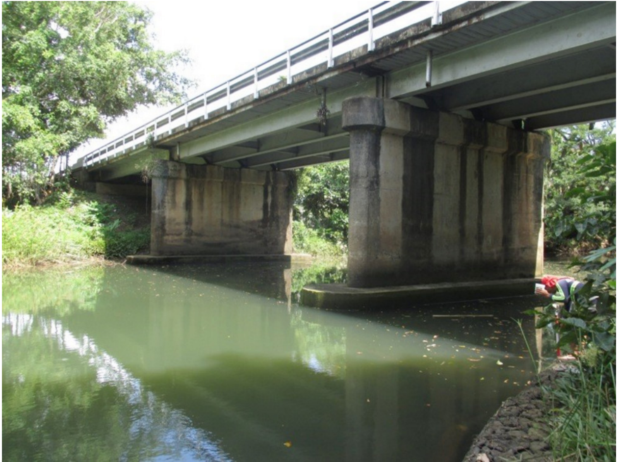
Figure 34. Upstream/downstream side of Bacungan Bridge
