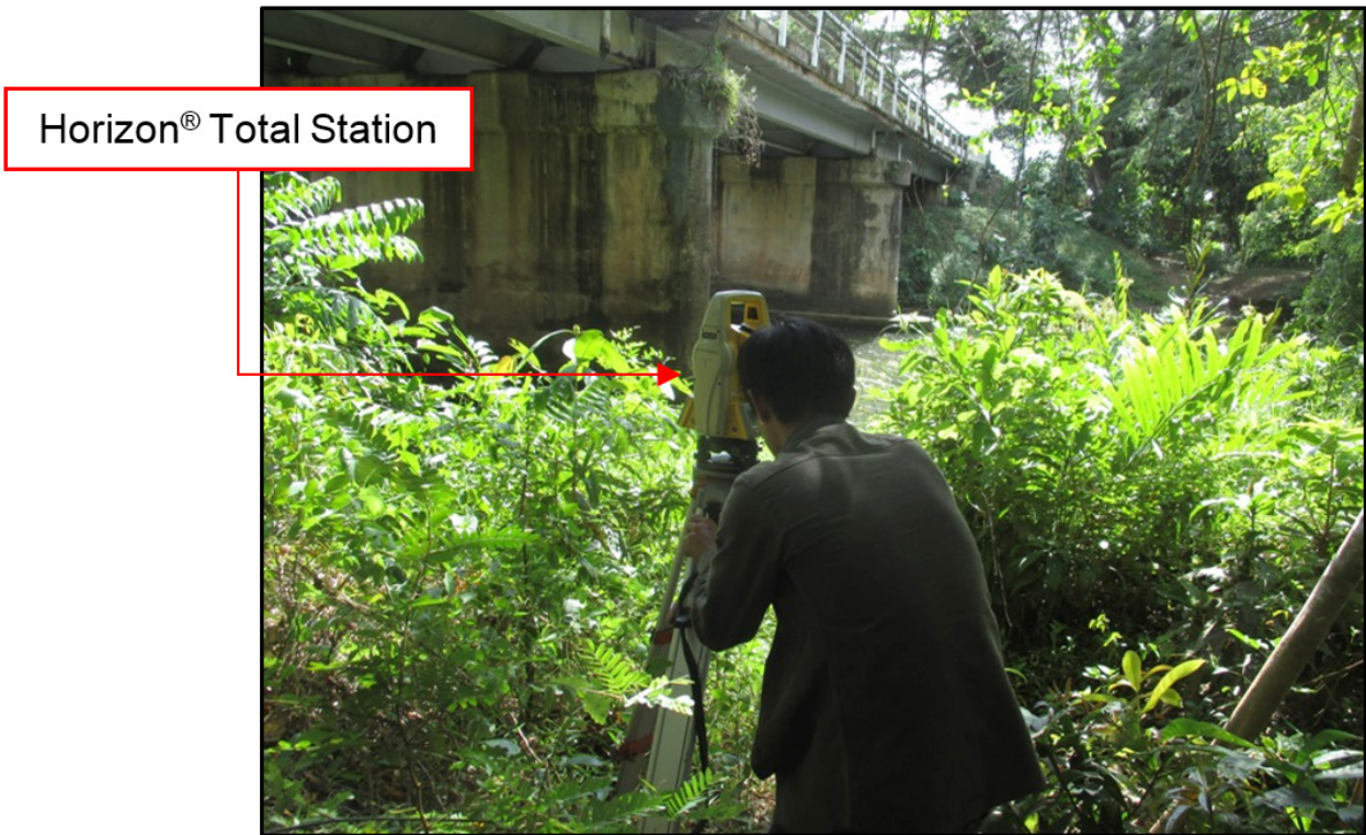
Figure 35. As-built survey of Bacungan Bridge
