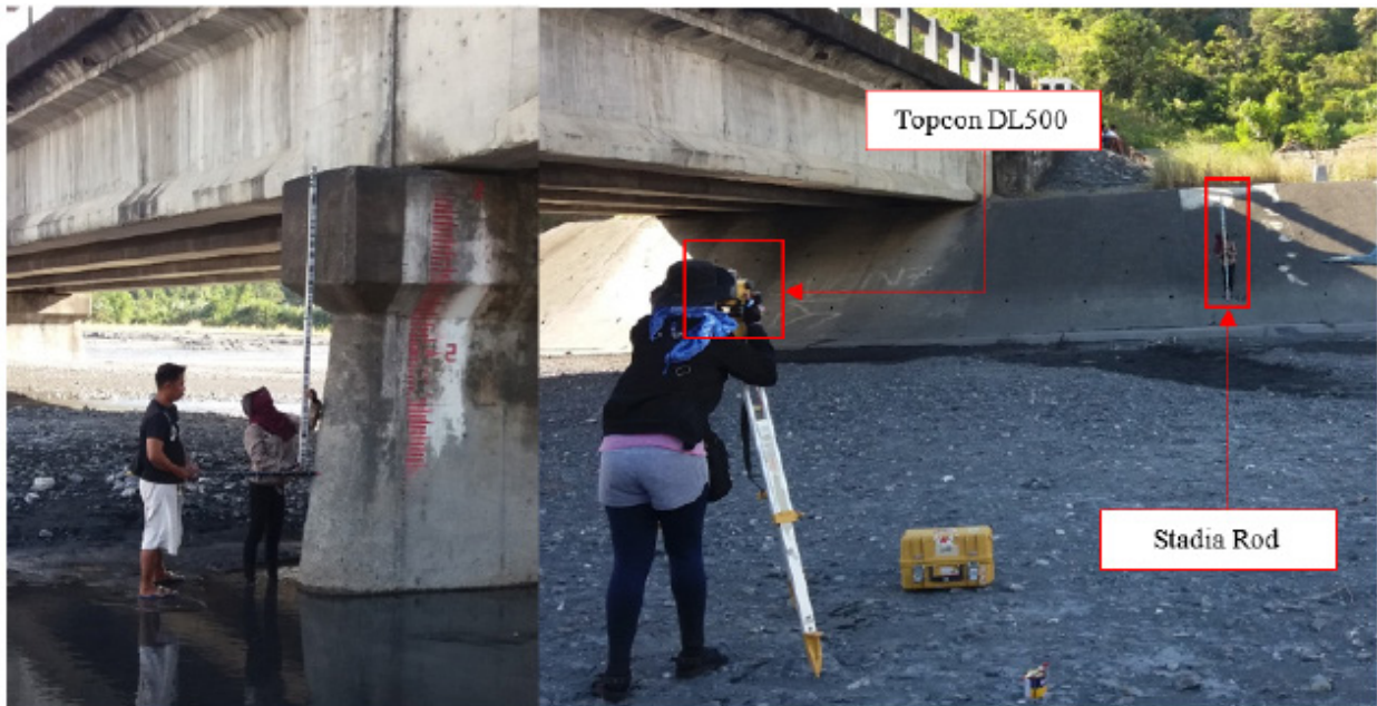
Figure 44. Water level marking at Amnay Bridge, Brgy. Pagasa, Municipality of Sablayan
