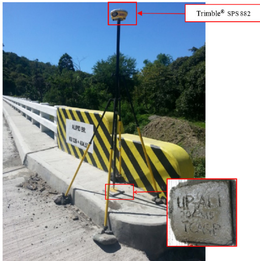
Figure 39. GNSS receiver set up, Trimble® SPS 882, at UP-ALI, Alipid Bridge approach in Brgy. Sto. Niño, Municipality of Sablayan, Occidental Mindoro
