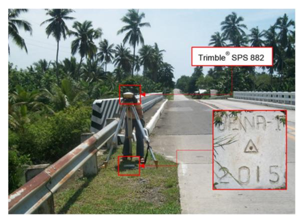
Figure 38. GNSS receiver set-up, Trimble® SPS 882, at UP\_INA-1, located beside the approach of Inagauan Bridge in Brgy. Inagauan Sub-Colony, Puerto Princesa City, Palawan.
