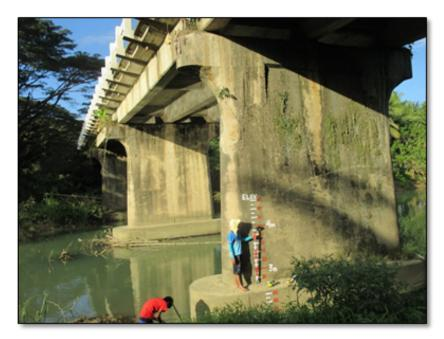
Figure 44. Water-level markings on Aborlan Bridge.
