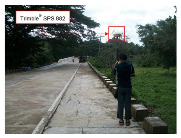
Figure 41. Gathering of random cross-section points along the approach of Aborlan Bridge.
