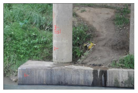
Figure 41. Water Level Mark at the pier of Tanao Bridge
