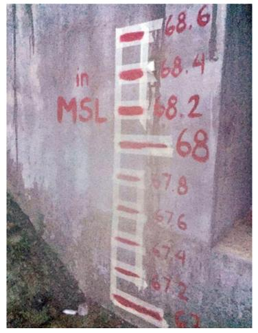
Figure 47. Water-level markings on the Baltazar Bridge
