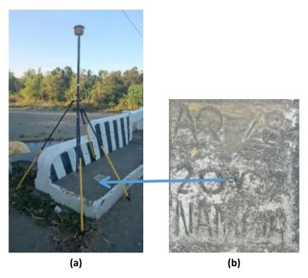
Figure 8. (a) GPS set-up over AQ-78, located at the NW side of the sidewalk of the Ipayo Bridge at Barangay Ipayo, Patnongon, Antique; and (b) NAMRIA reference point AQ-78, as recovered by the field team
