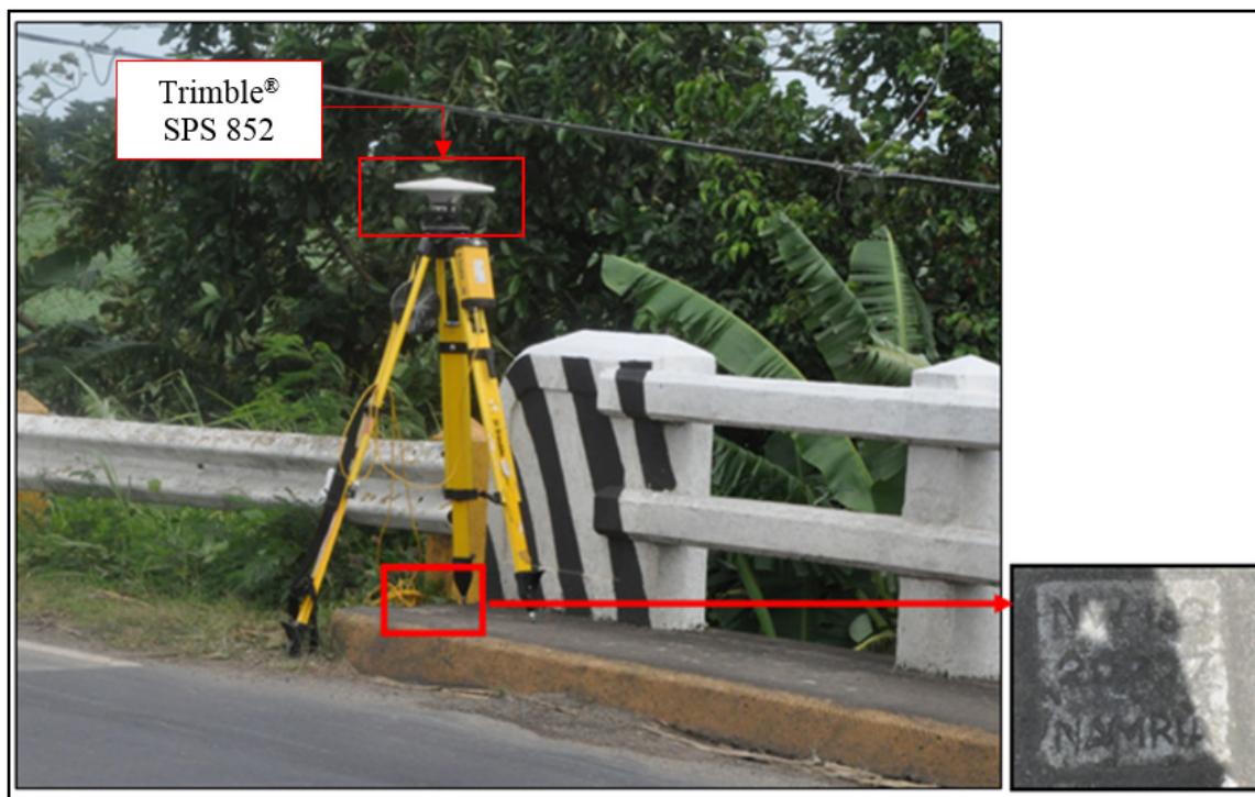
Figure 34. GNSS base receiver setup, Trimble® SPS 852, over NW-130 in Troso Bridge, Brgy. Daga, Cadiz City, Negros Occidental
