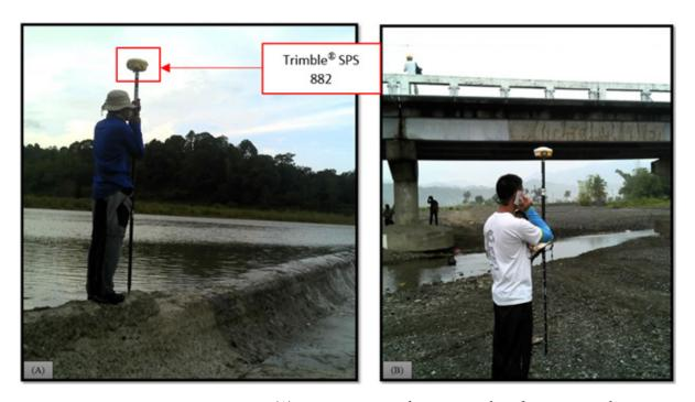
Figure 37. Cross section surveys (A) in Cangaranan Bridge, Municipality of Bugasong, and (B) in Valderrama Bridge, Municipality of Valderrama
