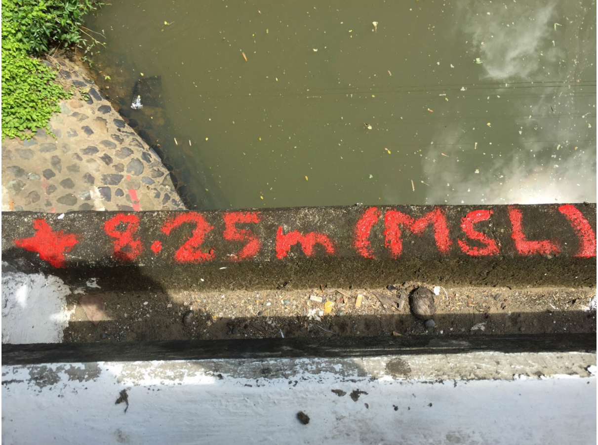
Figure 42. Water level markings on the cord of the Balantian Bridge
