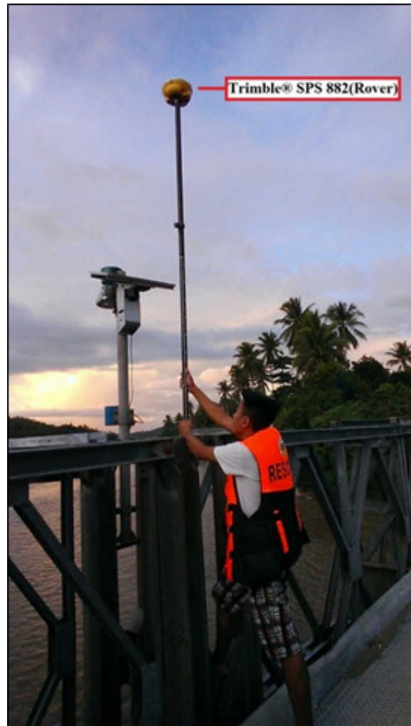
Figure 38. AWLS elevation acquisition at Guadalupe Bridge, Brgy. Poblacion, Municipality of Madalag
