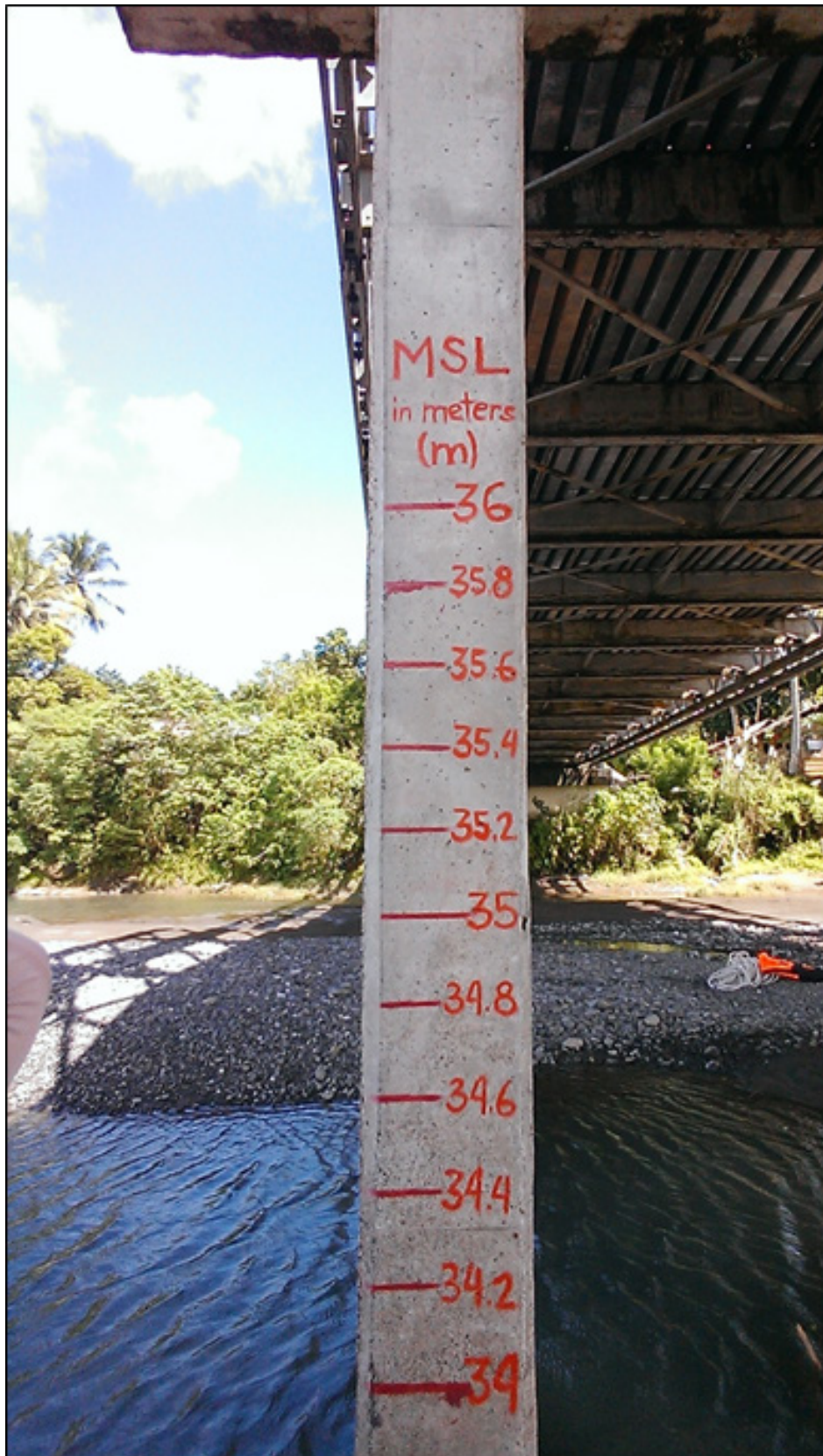
Figure 42. Water level gauge at one of the pier of Guadalupe Bridge, Brgy. Poblacion, Municipality of Madalag
