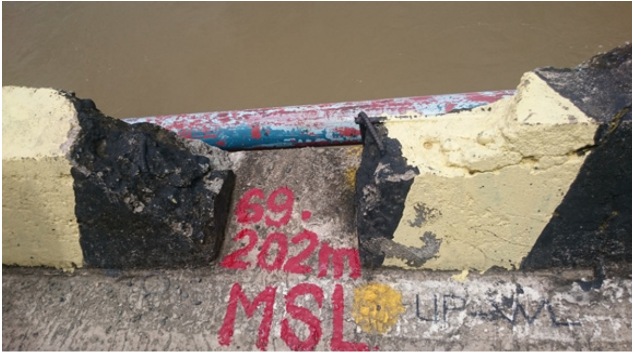
Figure 41. Water level markings on San Juan Bridge.
