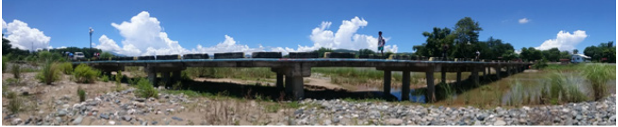
Figure 36. San Juan Bridge facing upstream.
