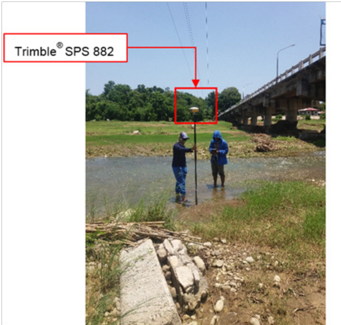
Figure 51. Manual bathymetric survey in Silay River
