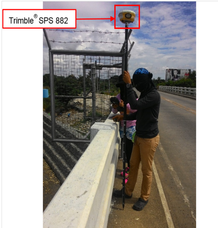
Figure 38. As-Built Survey of Burgos Bridge
