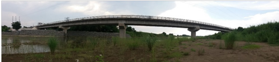
Figure 39. Sta. Maria Bridge facing upstream
