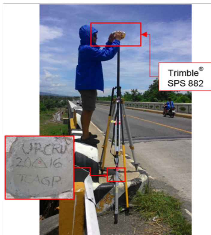
Figure 36. GNSS receiver setup, Trimble® SPS 882, at UP-CRU, located at the approach of Santa Cruz Bridge, in Brgy. Quinsoriano, Municipality of Santa Cruz, Ilocos Sur
