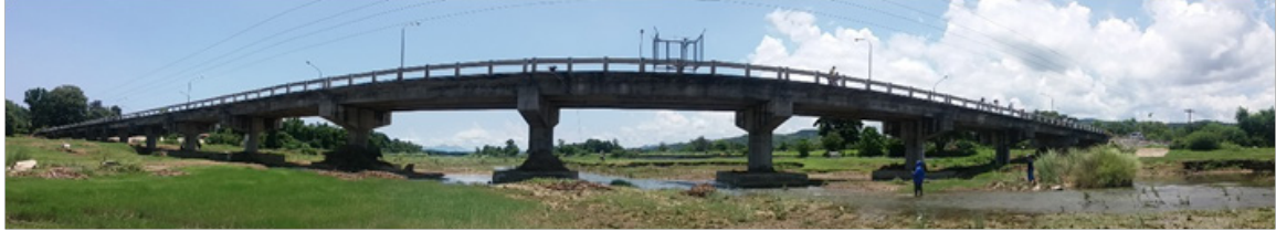
Figure 37. Burgos Bridge facing upstream
