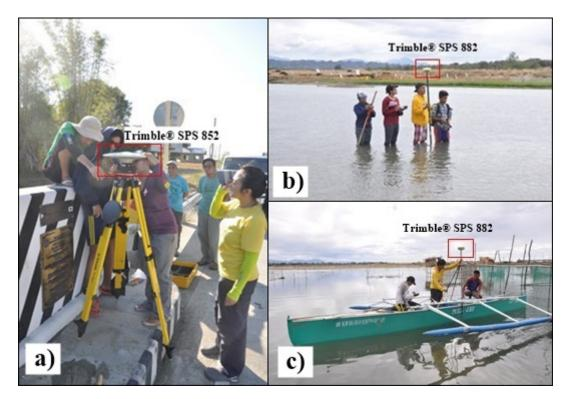
Figure 42.Bathymetric survey setup: (a) Base station at UP-SRT, (b) manual bathymetry at Laoag River, and (c) Bathymetry using echo sounder at downstream portion of Laoag River.
