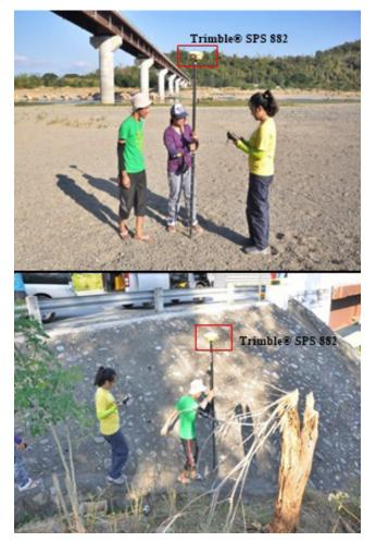
Figure 34.(a) Cross-Section survey at Sarrat Bridge and (b) conduct of the bridge as-built survey
