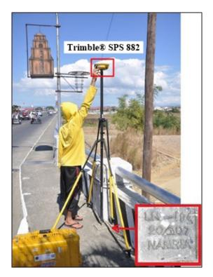
Figure 32.GNSS receiver setup, Trimble<sup>®</sup> SPS 882 at BM LN-184 on the approach of Gilbert Bridge in Brgy. No. 51-A, Nangalisan East, Laog City, Ilocos Norte.
