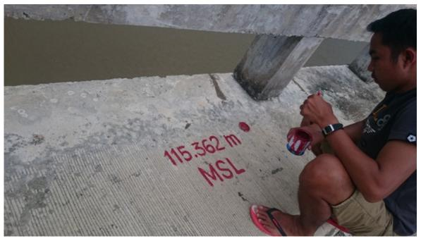
Figure 58. Water-level markings on Manabo Bridge
