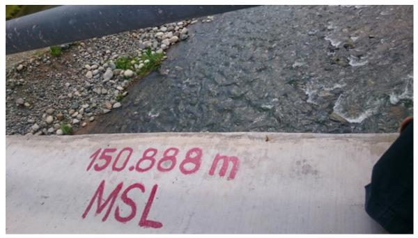
Figure 60. Water-level markings on New Ikmin Bridge
