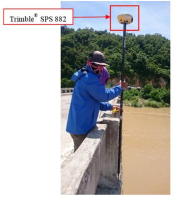
Figure 42. As-Built Survey of Manabo Bridge
