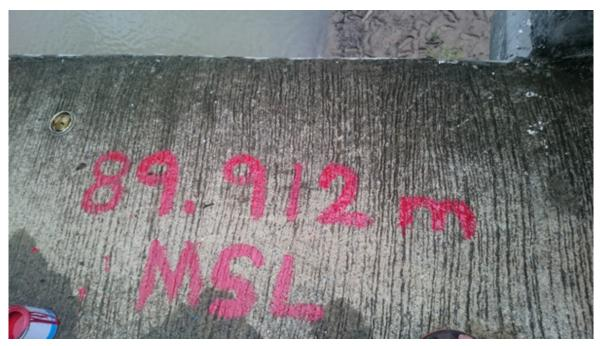
Figure 57. Water-level markings on Cervantes Bridge
