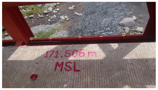
Figure 59. Water-level markings on Manicbel Bridge
