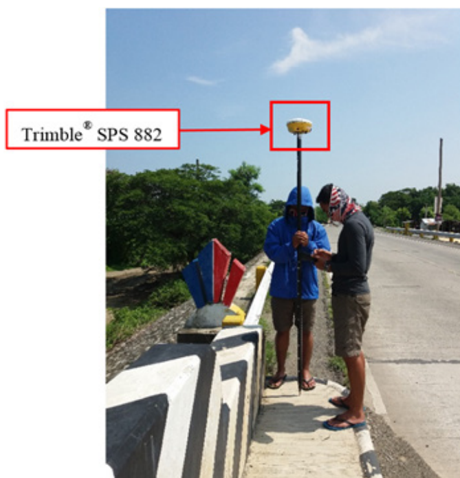
Figure 36. As-Built Survey of Santa Cruz Bridge
