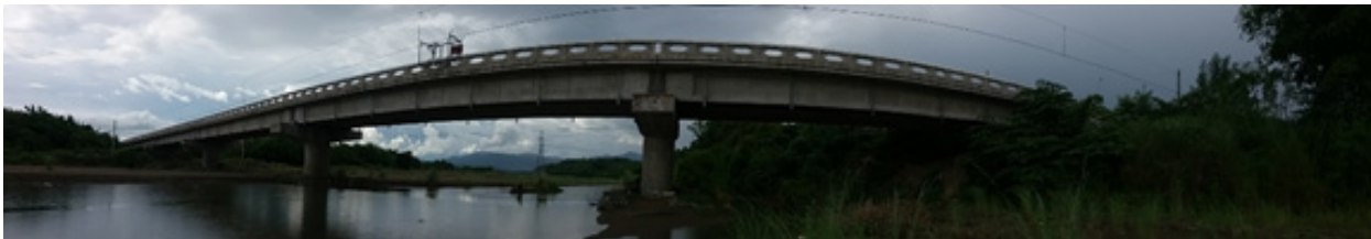
Figure 35. Buaya Bridge facing upstream
