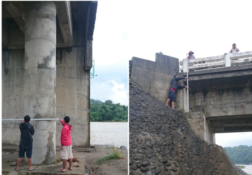
Figure 41. Cross-section survey at the Mamat-ing Bridge
