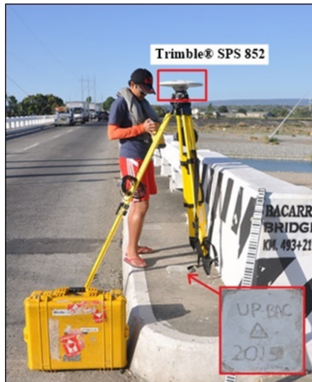
Figure 34. GNSS receiver setup, Trimble® SPS 852 at UP-BAC, Bacarra Bridge in Brgy. Buyon, Municipality of Bacarra, Ilocos Norte.
