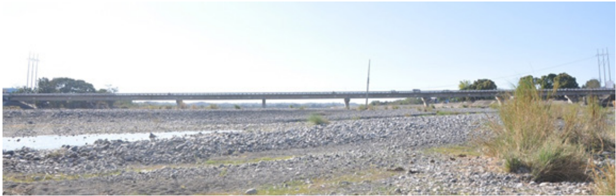
Figure 35. Quinonoan Bridge facing downstream
