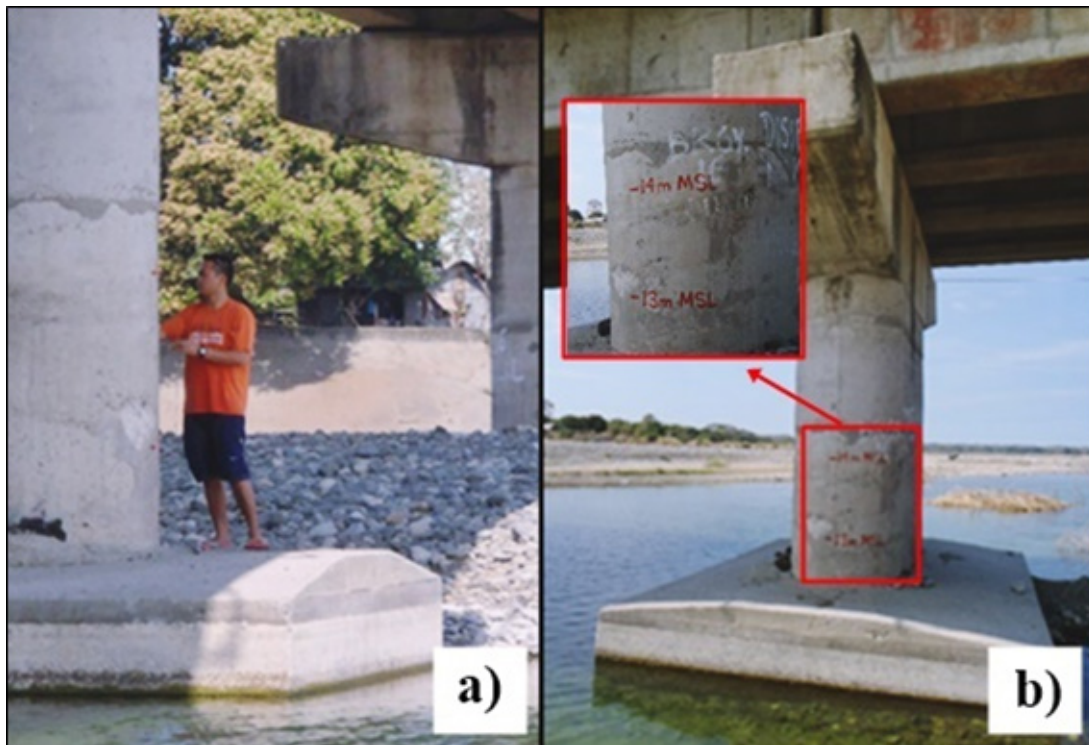
Figure 40. Water-level markings on Bacarra Bridge.
