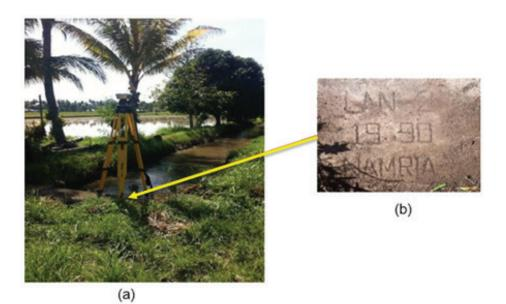
Figure 3. GPS set-up over LAN-02 on top of a concrete irrigation canal water gate in Brgy. Pinoyak, Lala, Lanao del Norte (a) and NAMRIA reference point LAN-02 (b) as recovered by the field team.
